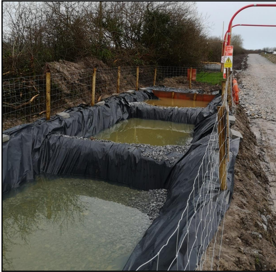
Figure 3-3 Multi-tiered settlement pond with stone filter
